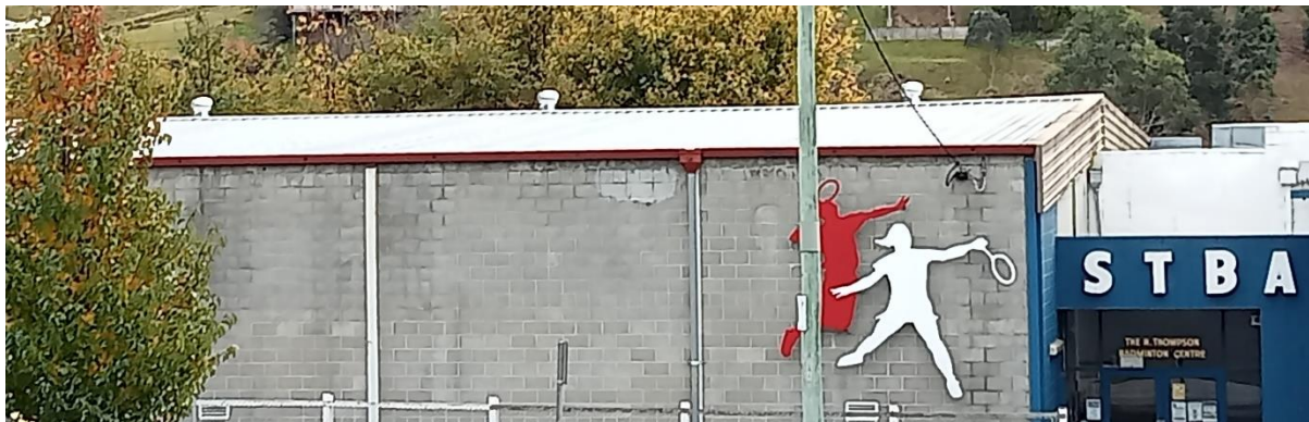
Image 1 The whirley birds installed on the roof of the hall
